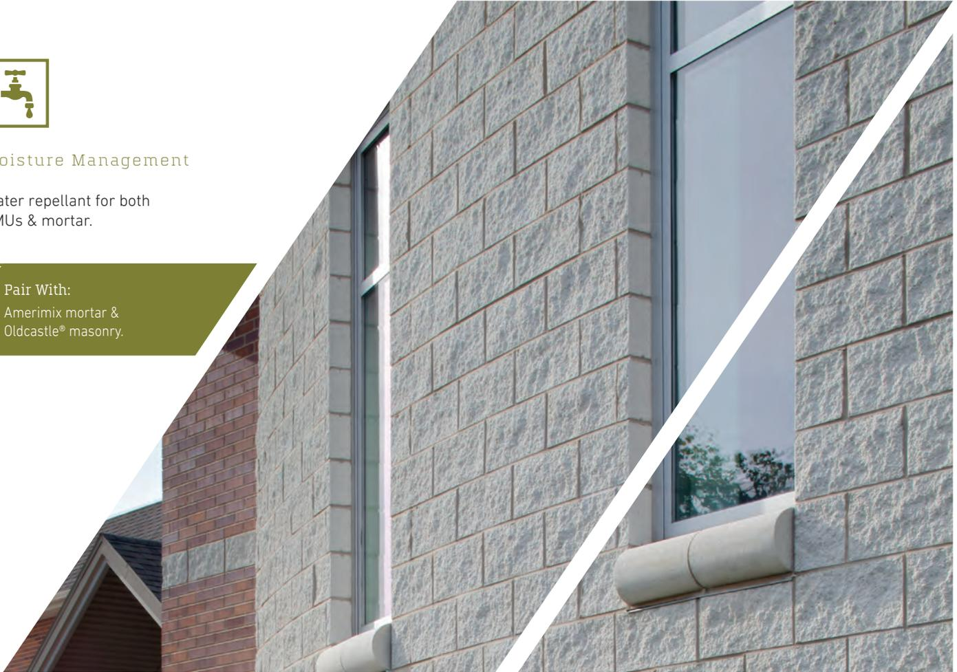
RainBloc® GP is a patented technology that can be added to mortar or concrete masonry block during the blending phase, which hinders water from penetrating the structure. This specially engineered formula creates a moisture barrier that will last the life of the building.
